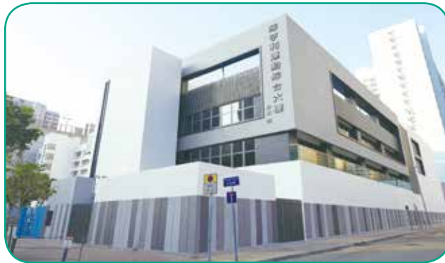
陳亨利運動綜合大樓建成。 The construction of Henry Tan Sports Complex was completed.
